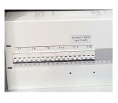
There is ample DIN space in the board to accomodate tenancy main switchs outgoing circuits.
